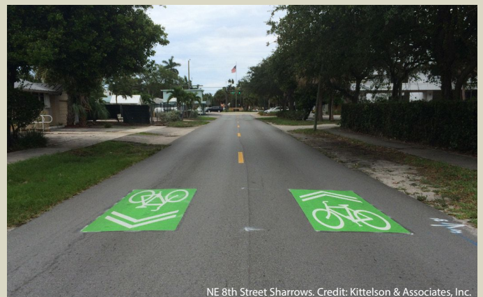
NE 8th Street Sharrows. Credit: Kittelson & Associates, Inc.
