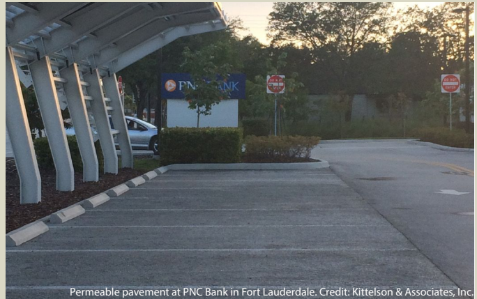
Permeable pavement at PNC Bank in Fort Lauderdale. Credit: Kittelson & Associates, Inc.
